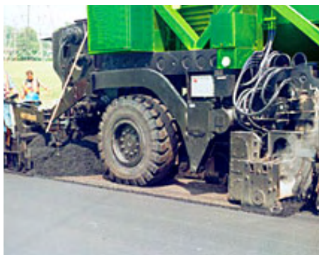
Image 30. Reclaimed asphalt paving
