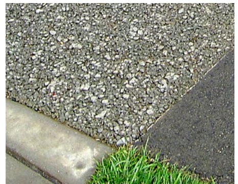
Image 28. Pervious asphalt
